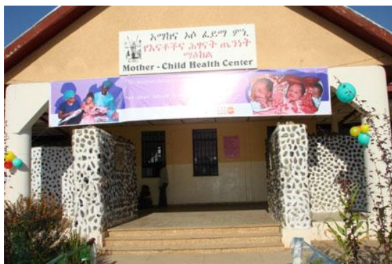
Mother - Child health centre installed by KMG Ethiopia at Durame, the capital of Kembatta Tembaro Zone. Source: www.kmgselfhelp.org
